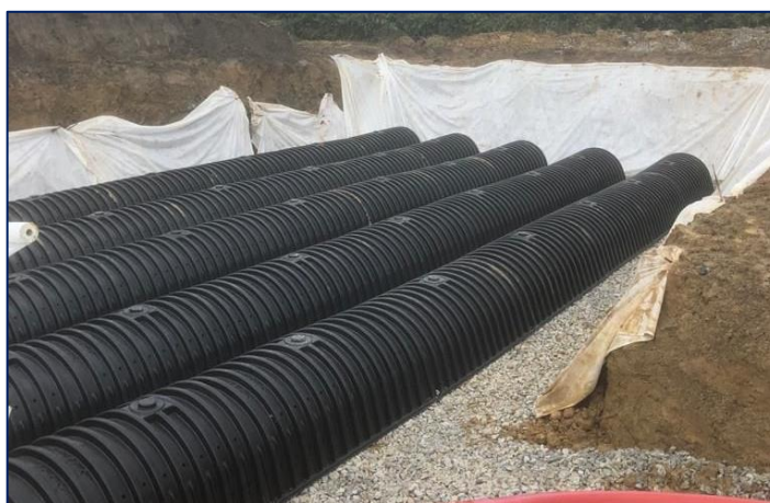
Figure 3.8 – Typical Poly-Tunnel Installation Arrangement
